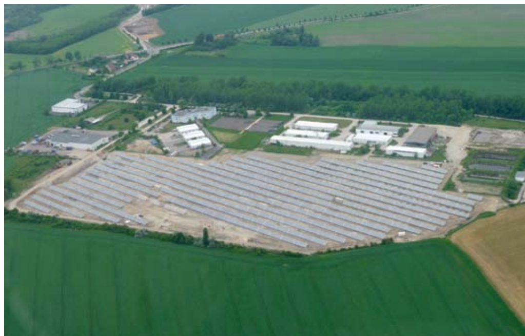
Power plant Blumroda
